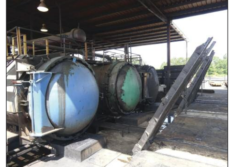
Operating three creosote cylinders 80 ft. x 8 ft., 72 ft. x 8 ft., and 140 ft. x 8 ft....
