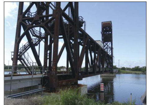
Railroad Bridge is only 1.25 million pounds shown in the up and down position.
